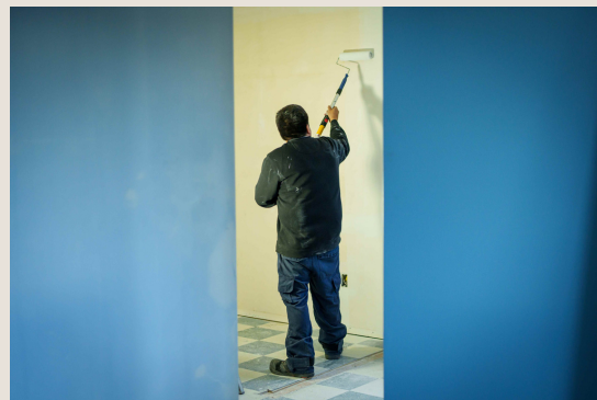
Renovations being done in Tl'etinqox
