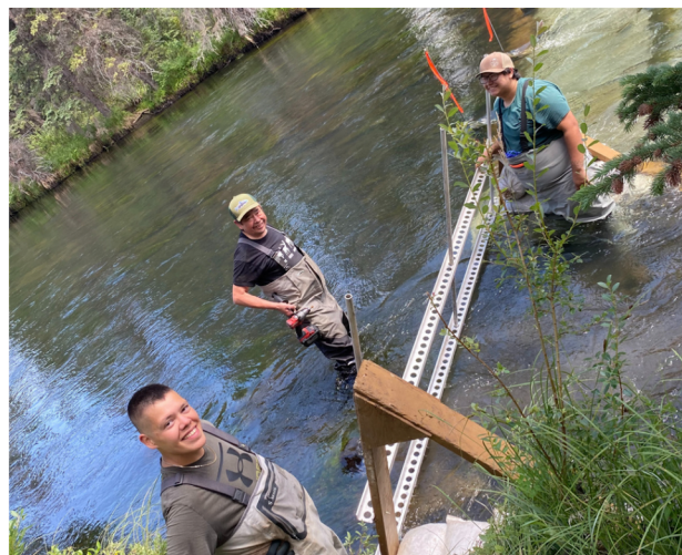
TNG Fisheries Technician Winston Bambrick with UFFCA technicians Carl Siwallace and Brendan Wright installing the brood collection fence for emergency enhancement of Upper Chilcotin Jās.
