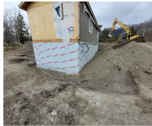
Photo 3: Backfill starting on a foundation in Xeni
