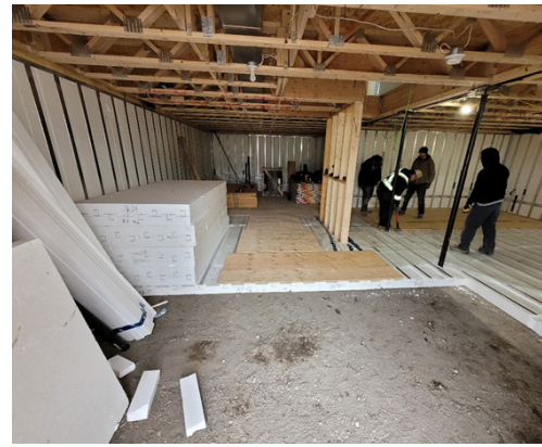
Photo 1: Styrofoam and steel floor system that replaces concrete
