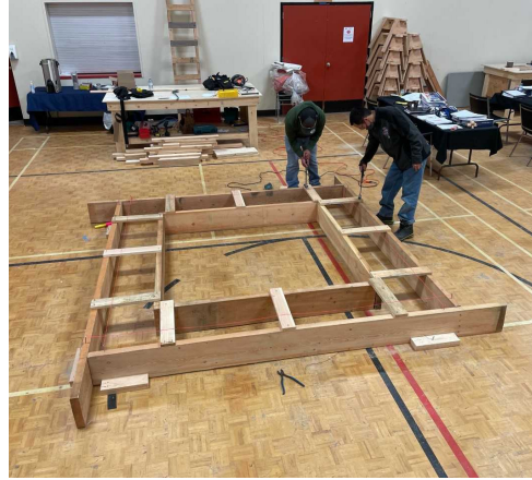
Photo 1: Footing Formwork
