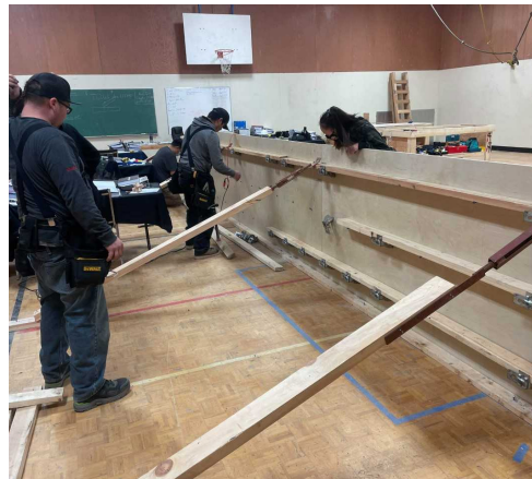
Photo 2: Footing Bracing
